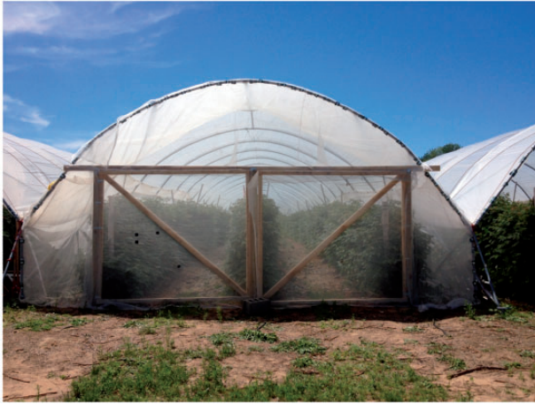
Fig. 1. High tunnel raspberry planting with netting added to exclude D. suzukii . The barn style wooden doors were installed to allow access for a tractor-pulled sprayer.
